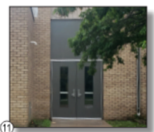
11 HOLLOW METAL STOREFRONT DOORS & HOLLOW METAL FRAME
