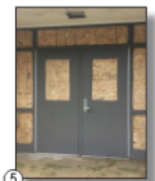
5 HOLLOW METAL STOREFRONT DOOR & HOLLOW METAL STOREFRONT FRAME
